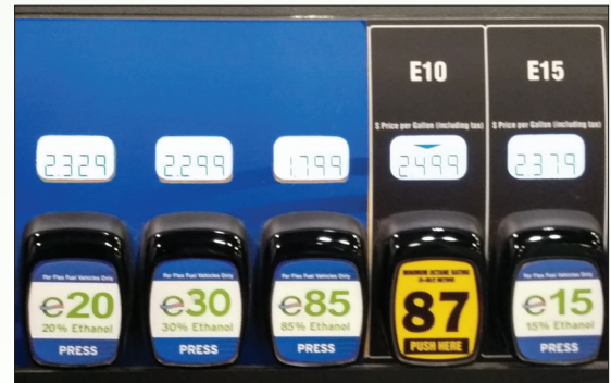
DIAGRAM 2. E10 and E15 can be sold from same hose with proper labeling..
